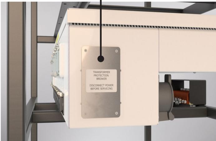
Remove the cover plate to access the breaker and set breaker to ON position
